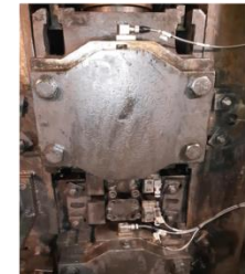
Front view of rollers
